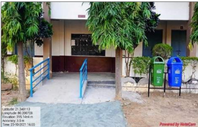
Ramp For Chemistry Laboratory and Main Building
