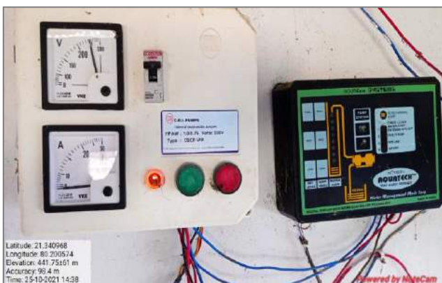
Control panel for water supply
