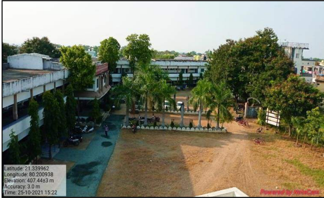
View of Main Building and Entrance
