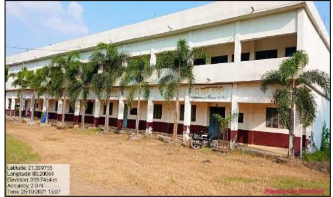
Class Rooms In New Building
