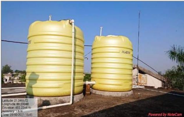
Water Tanks on Terrace
