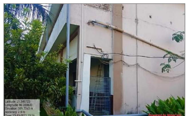
Rain water Harvesting
