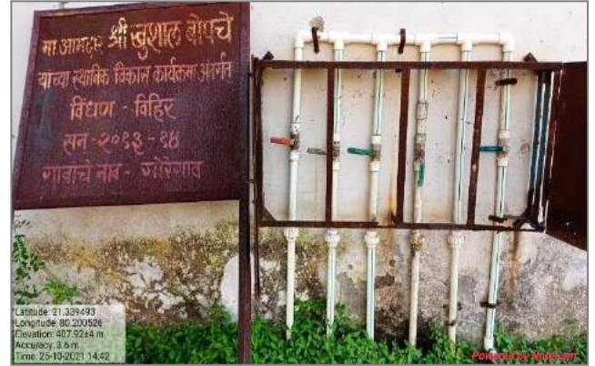
Valves Controlling the water supply to Different Buildings
