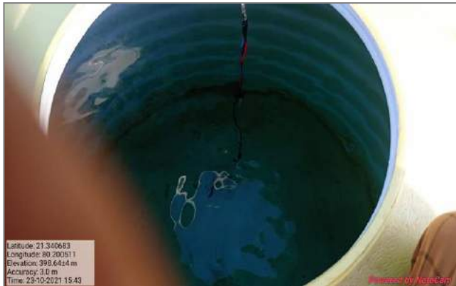
Sensor System In Water Tank
