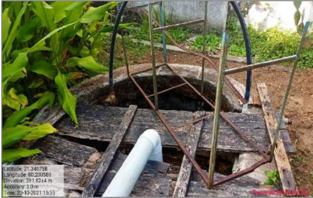
Rain water carried in Well
