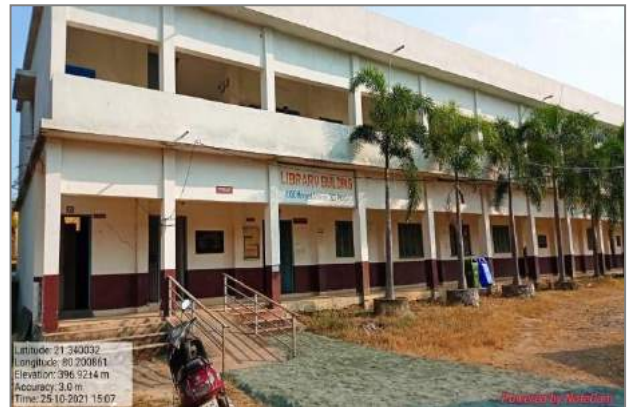
Ramp facility For Library
